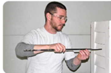
Remove SnakeBit and Leave Wire in the Wall
