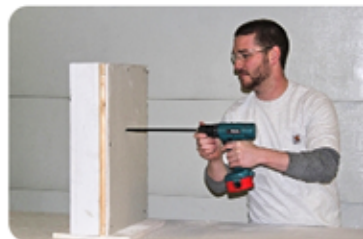
Drill Through the Wall
